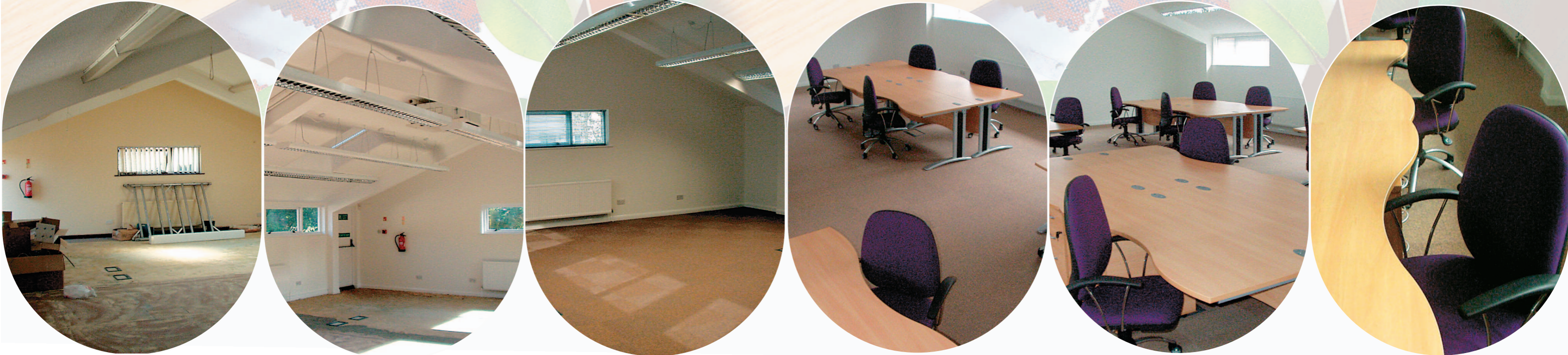
Photographs show the progress of the office conversion
